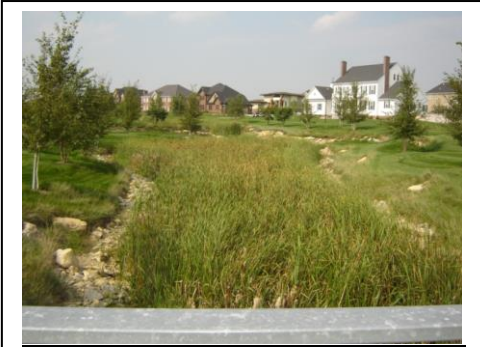
Example of a Drainageway or Surface Drain
