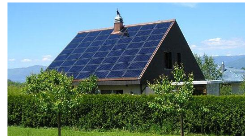
Example of a Solar Conversion System, Structure-mounted
