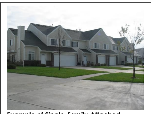
Example of Single-Family Attached
