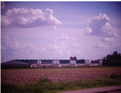
Example of an Animal Confinement Building
